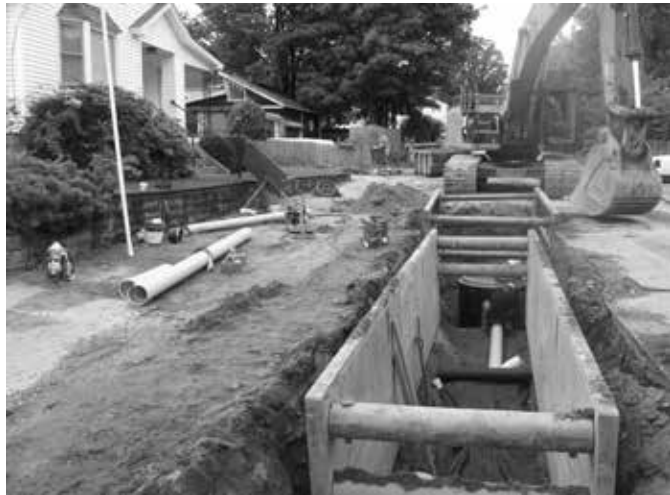
2016 Sewer Replacement Project, Warren Ave
