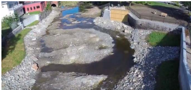
With the dam removed, the river is now free-flowing
