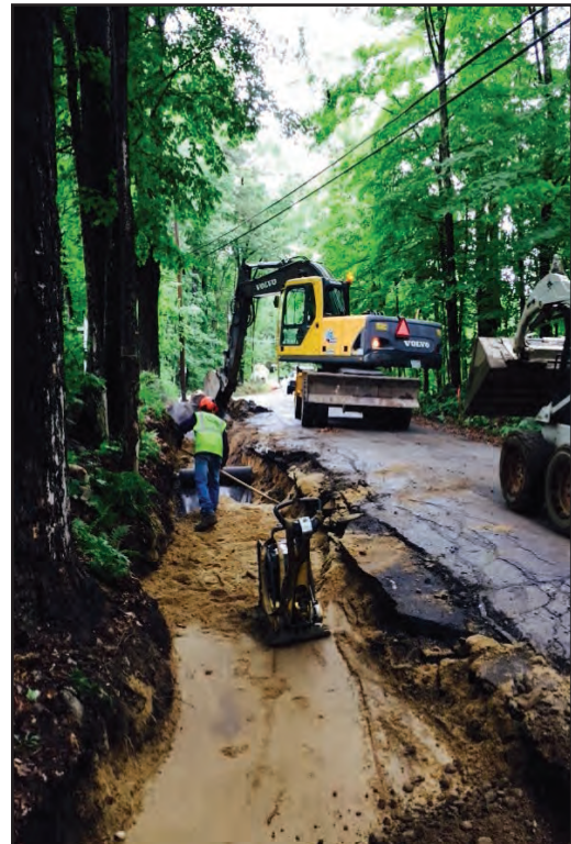
Drainage work on Paige Hill Road
