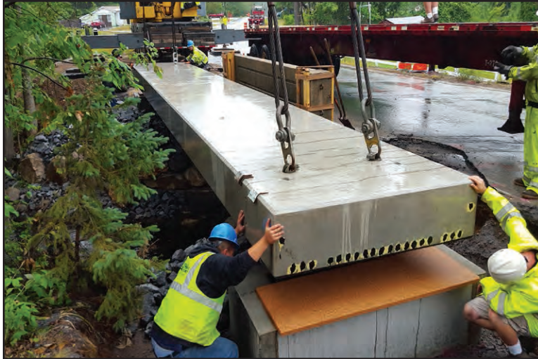
Pedestrian bridge installed at New Boston Road
