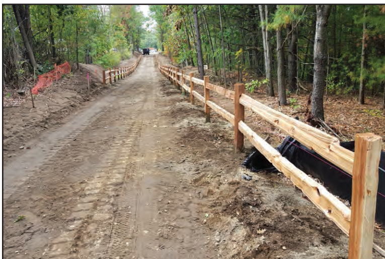
Pedestrian bridge installed at New Boston Road
