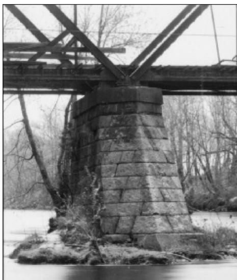
Detail of pier upstream nosing, showing stonework. Looking southeast.
