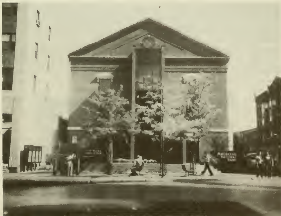
Downtown revitalization gets a boost through renovation of the Goodwill building into "City Plaza"
