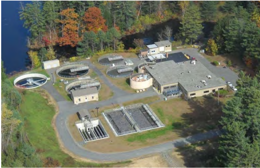
Facility aerial view
