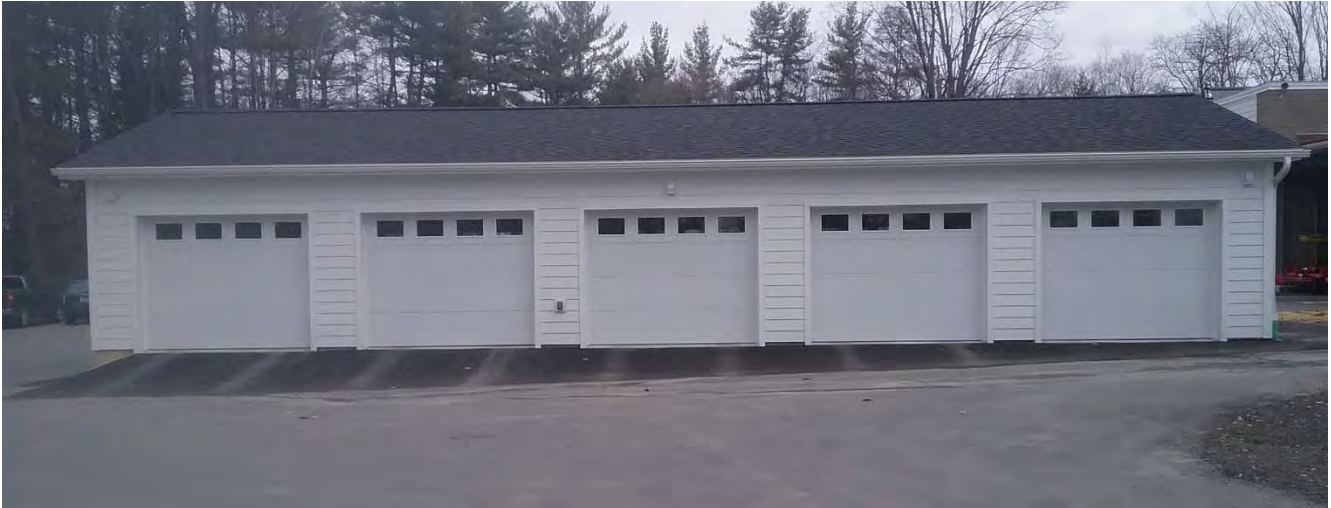
Pass-through garage at the Police Department
