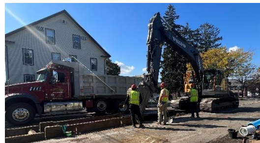
Sewer Pipe Installation by N. Granese & Sons along High Street
