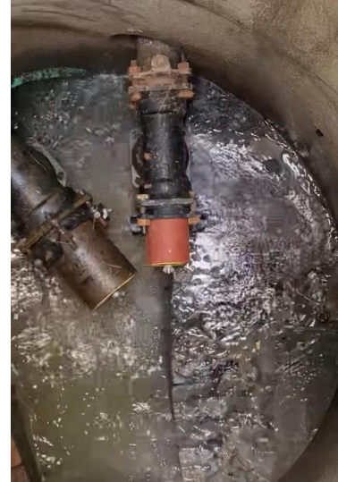
Sewer Manhole Repair
