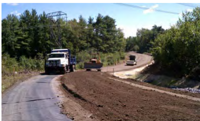
Geotextile Installed Under Reclaim
