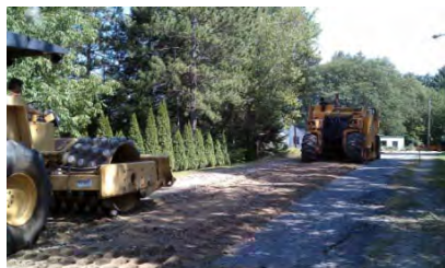
Reclaimer Grinds Old Pavement
