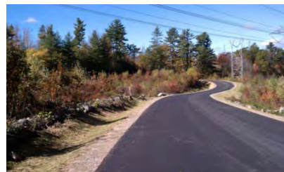
Base Asphalt Installed Over Reclaim
