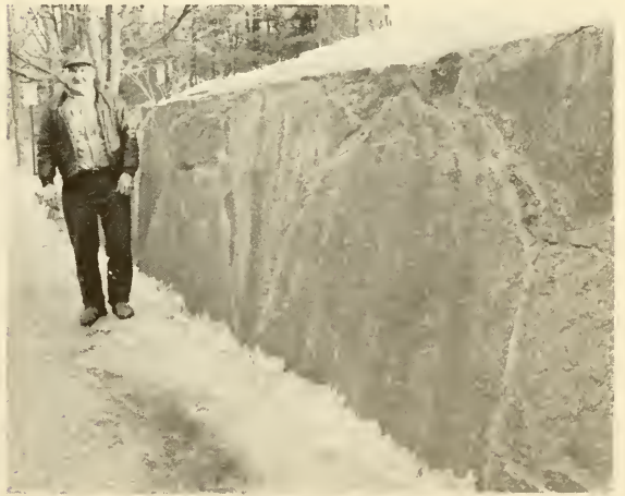
Wall on Mill Road
