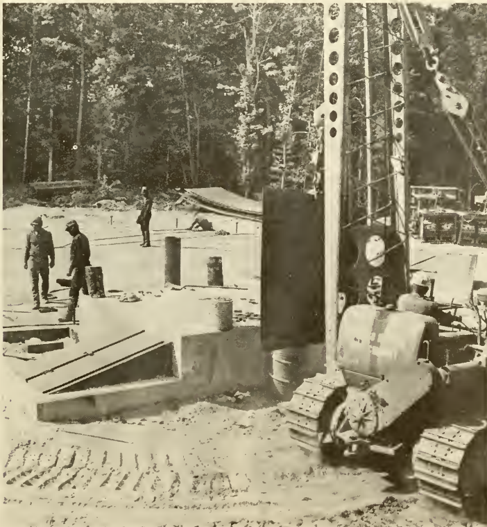
Foundation of New 3.2 Million Gallon Water Standpipe
