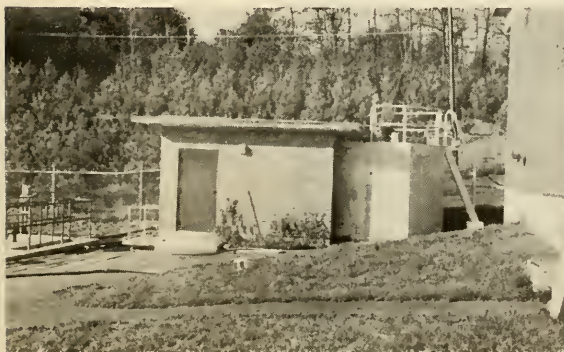
GREASE HANDLING FACILITY NOW IN OPERATION.
