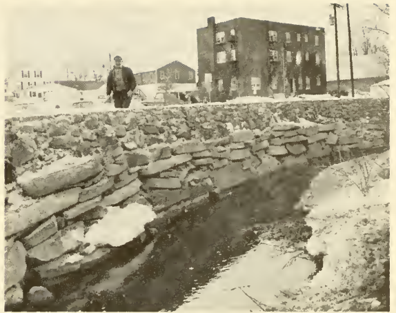
Wall at Pettee Brook
