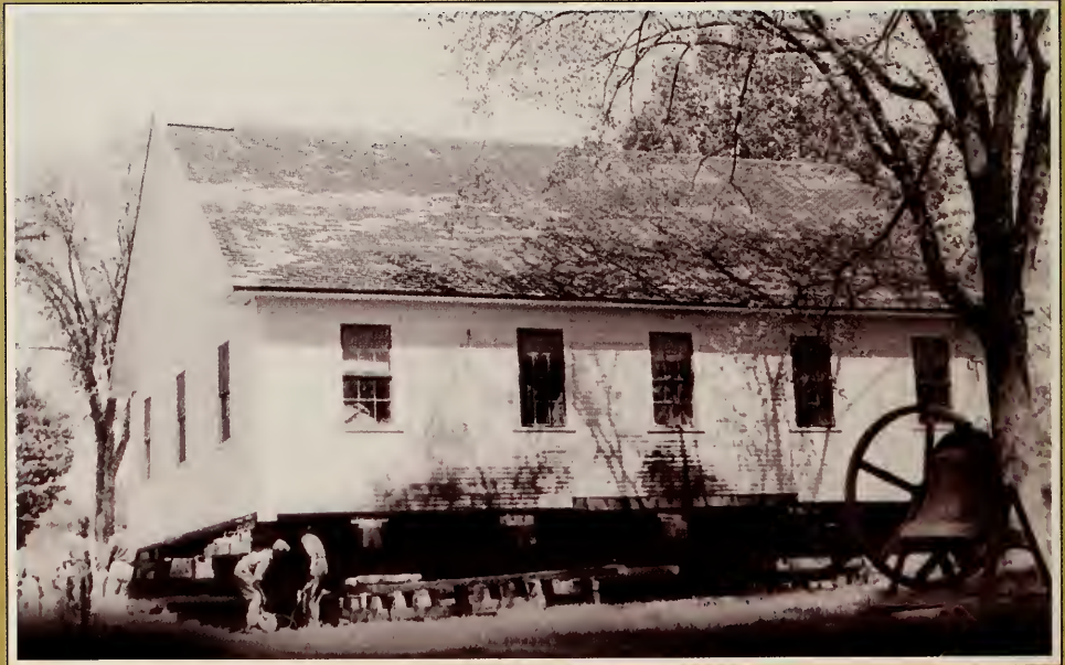
Jacking up Town Hall for moving, May, 1947.
