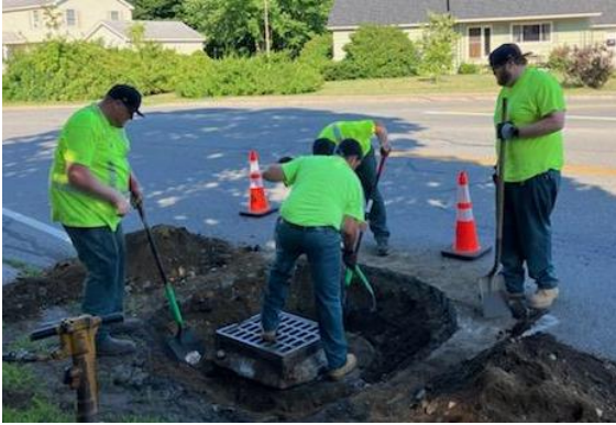
Sewer and Drain Division Repairing a Catch Basin
