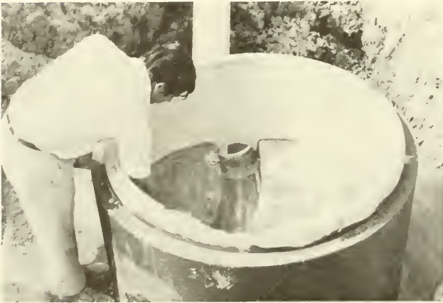
Public Works Director George Crombie Inspects Properly Constructed Manhole
