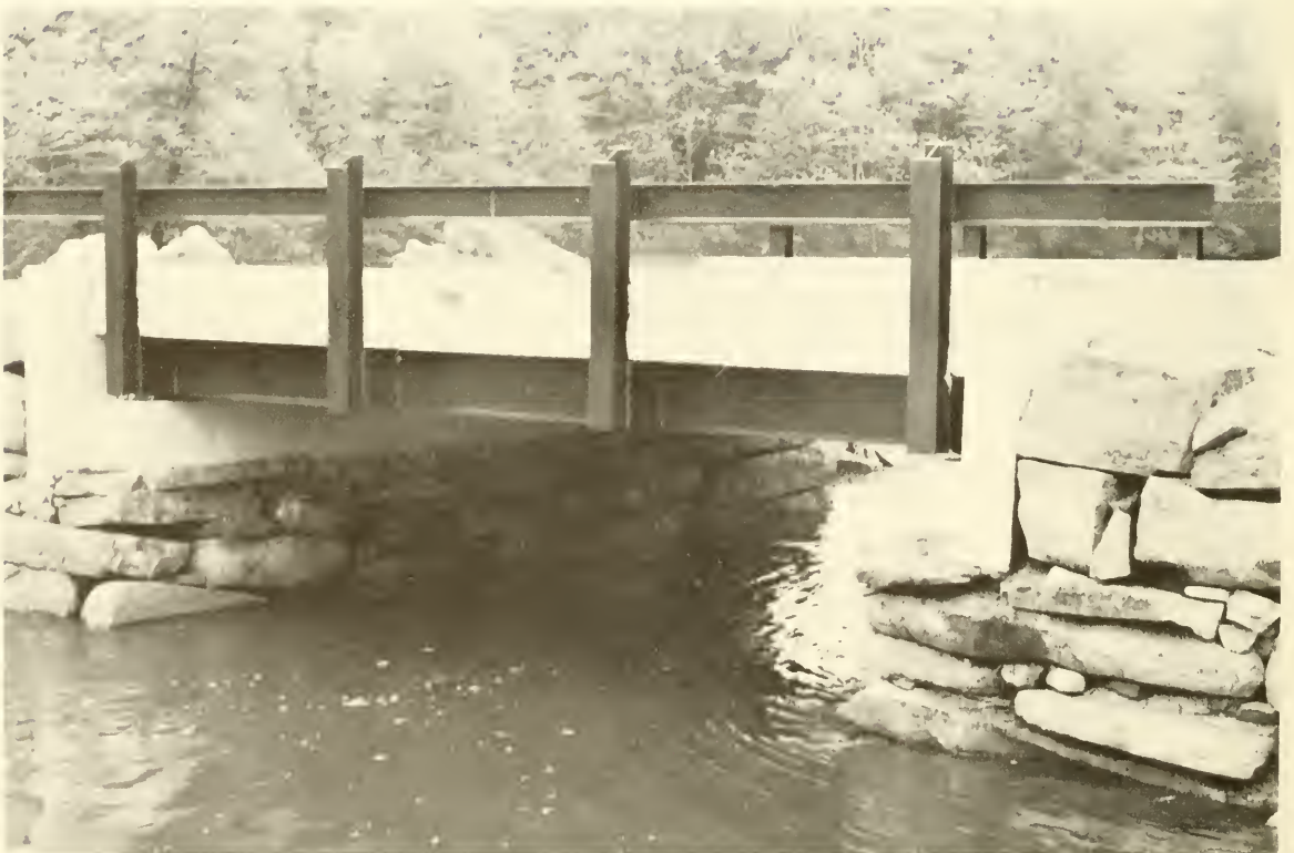
Crommet Creek Reconditioning Completed
