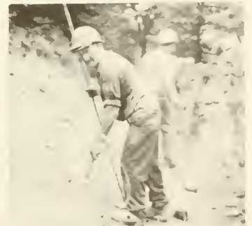
Rudy Niemi Loading Holes in Preparation for a Blast
