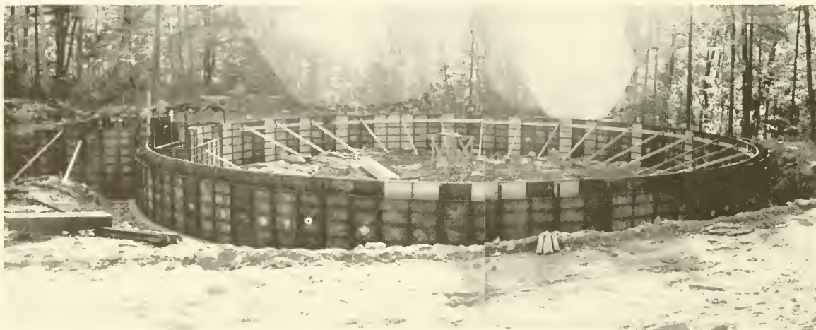
Construction of New Four Million Gallon Water Tank - Foundation
