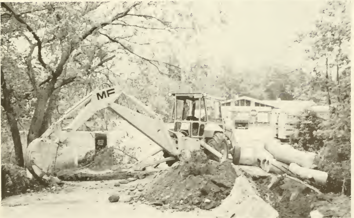
New Drainage for Bay View Road
