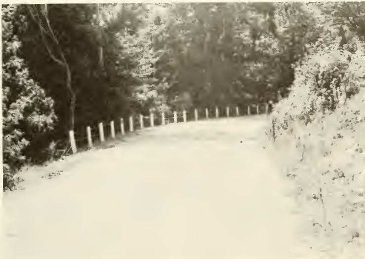
Guard Rails along Bennett Road were Replaced by C. Fogg, Jr. & Crew
