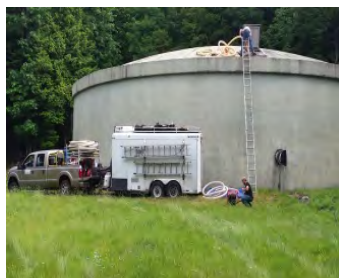
Divers cleaning Sand Hill Tank
