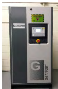
VSD air compressor
