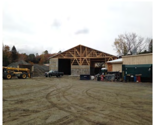
New Winter Maintenance Storage Facility
