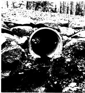
Per repair / replacement guidelines from NH Emergency Management, the storm damaged and failed 48" culvert was replaced with a 72" design. The work was put out for competitive bid and completed with a \$98,000 price tag.
