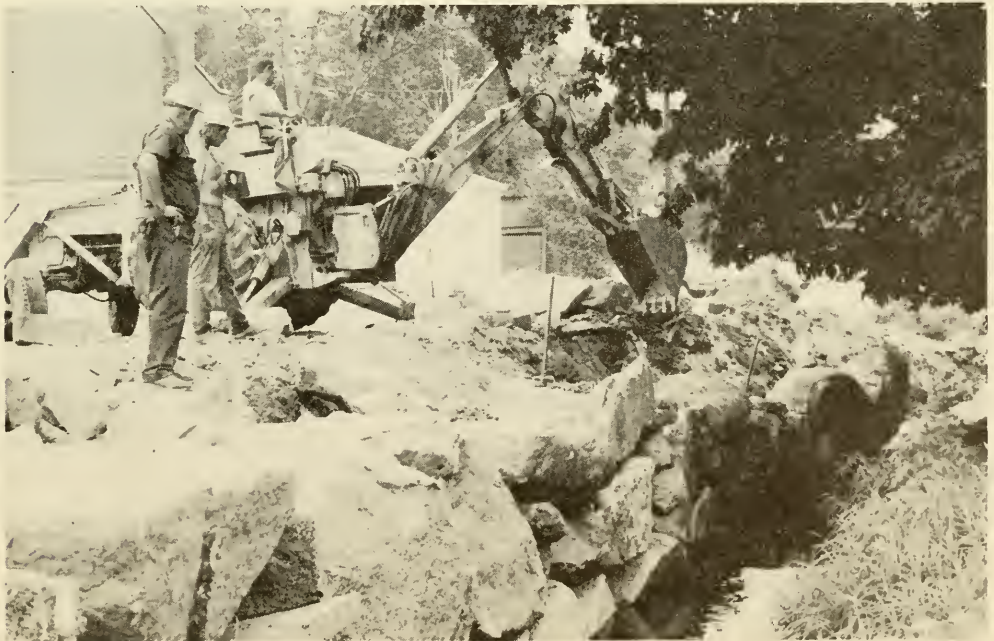
Granite wall construction at end of Jenkins Court
