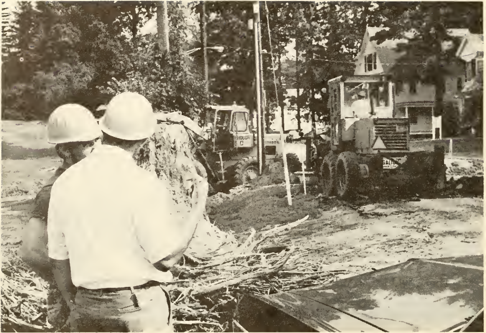
Assistant Public Works Director George Crombie Directs construction at Ballard Street
