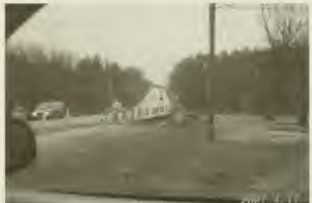
April 2007 flooding on Route 101
