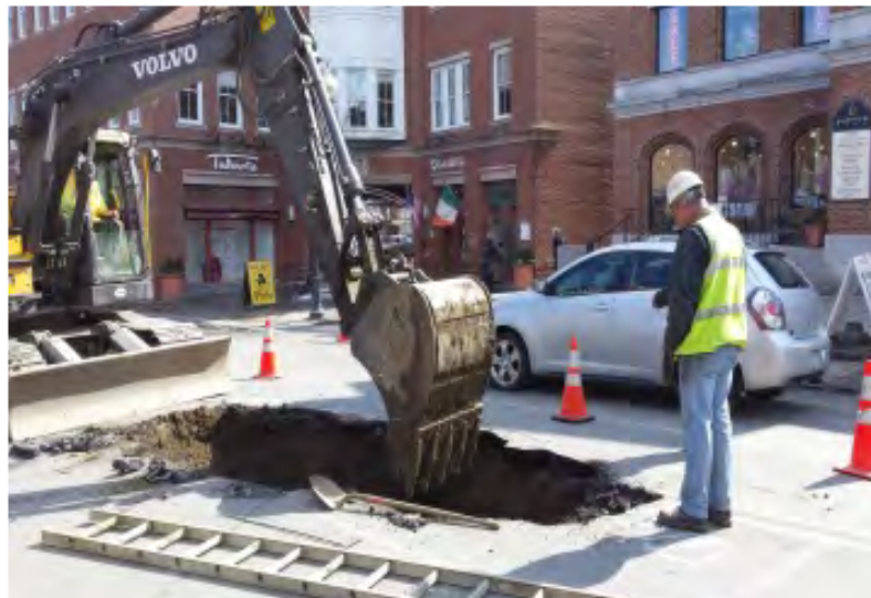
Repairing 1893 water main
