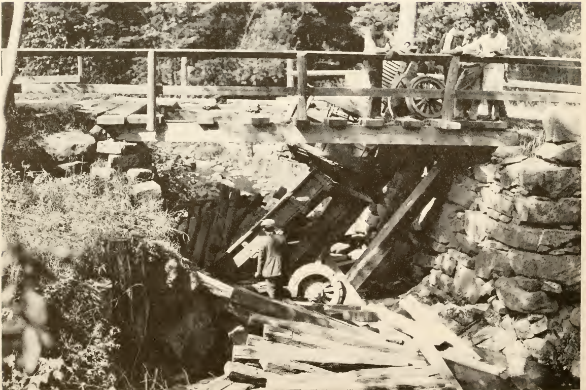
Picture taken around 1925. A State highway truck carrying old railroad ties was a bit much for former Oyster River bridge on Mill Road
