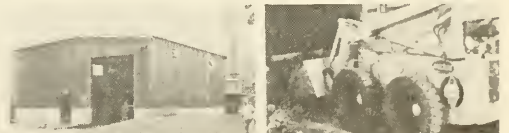
A small metal building encloses the charging floor. Trucks dump the refuse just inside the large door.
