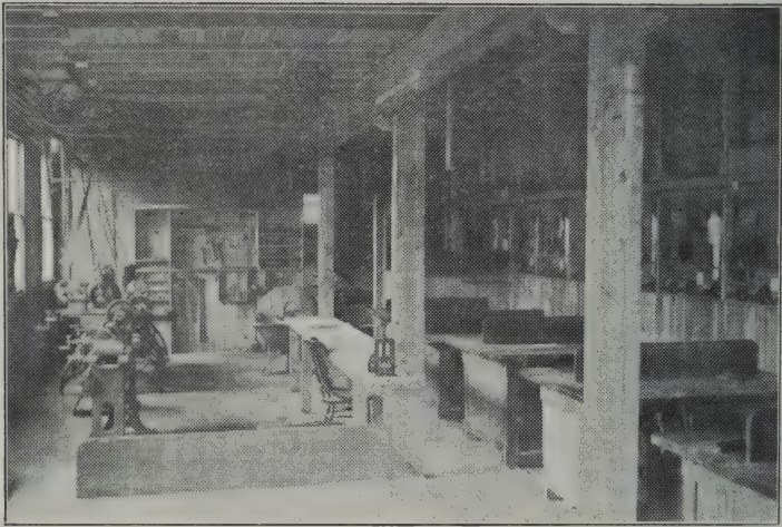
CUT No. 10—MACHINE ROOM.
