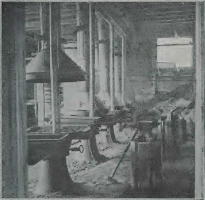
CUT No. 9—FORGE ROOM.
