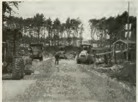
County Road Reconstruction Bedford High School/Middle School
