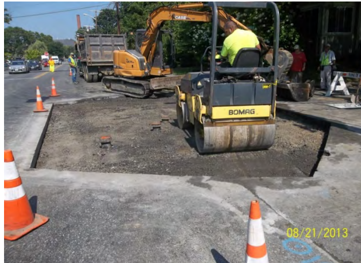
Preparing to pave at Summer Street
