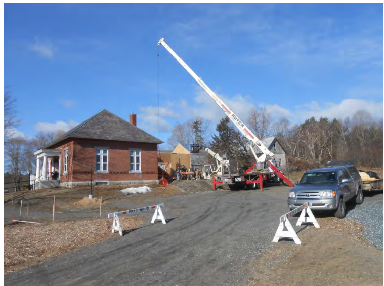
Construction of new addition – Summer 2013
