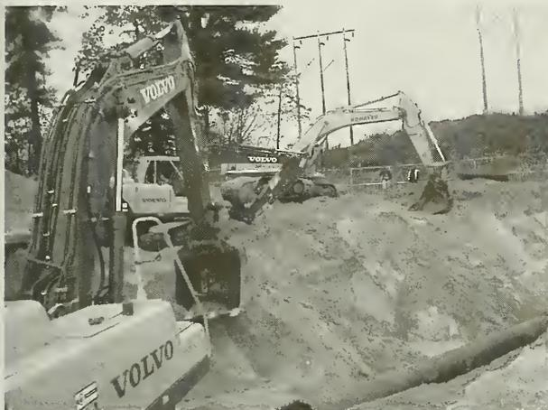
the Mother's Day flood and the landfill back together after the October 2005 flooding. Over the course of the winter we worked on the landfill cap to make the necessary repairs to the landfill downchutes and outfall pipe. This project took several months to complete but the work was done mostly by our in-house staff using rented or town-owned equipment. If not done in-house, this was a
