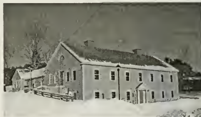
(132 Bedford Center Road)
