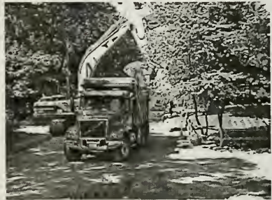
(Ministerial Road Construction)
