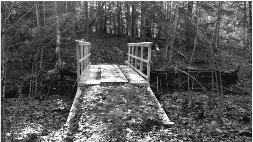
New bridge installed by the Society for the Protection of NH Forests to reduce creek erosion on the town owned Schreiber property. Part of the Powder Major trail system.
