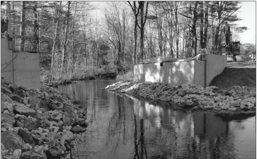
New bridge abutments at the Nute Road Bridge over the Bellamy River.
