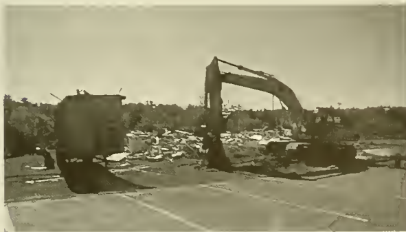
(Town Pool Under Construction)
