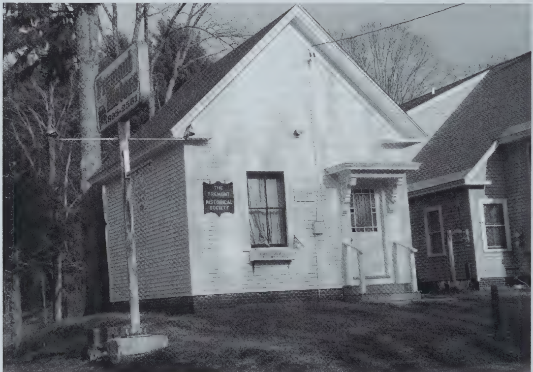
Historic Building at 282 Main Street Freshly painted and reroofed in 2015
