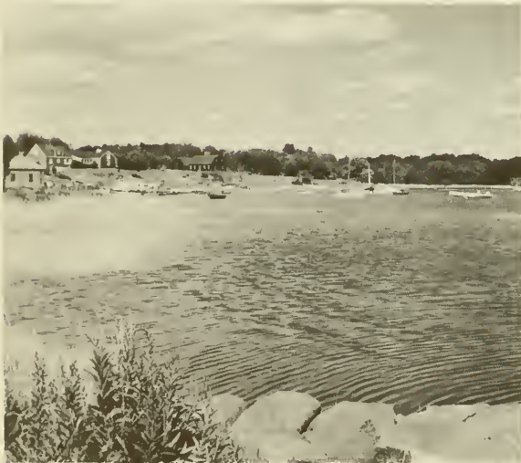
Oyster River from Shipyard Landing. The office - restroom building is on the extreme left.
