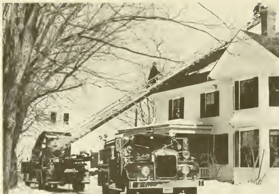
A chimney fire at Highland House in January, 1967. The Durham—UNH Fire Department is using the 75-foot aerial ladder. In the foreground is the 1,000-gallon-per-minute pumper.
