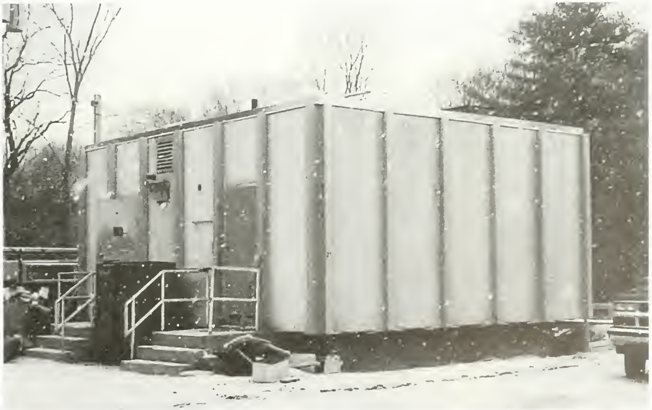
Webster Avenue Pumping Station
