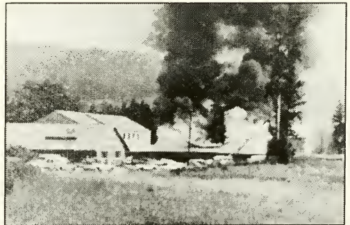
The IGA store fire at Campton Plaza
