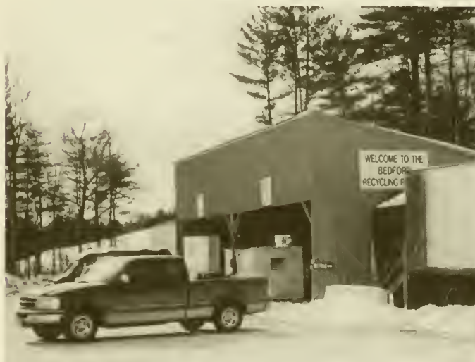
Bedford Transfer Station: Re-cycling Center
