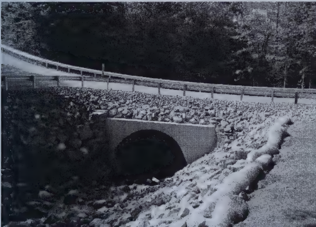
Basin Bridge after reconstruction by NH DOT
