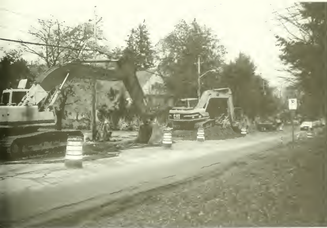
Sewer Separation Project – Court St.
