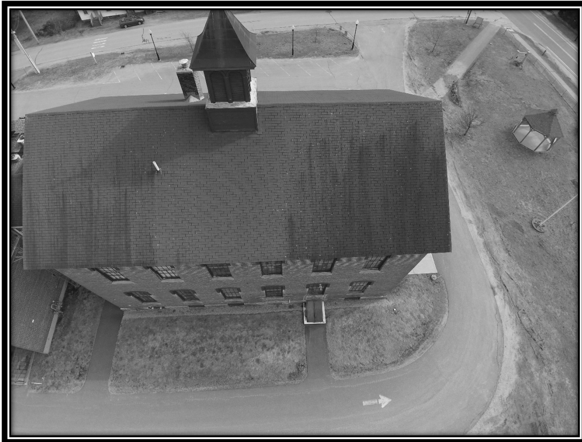
Mike Bradford took this picture with his drone to inspect the shingles on the roof of the Municipal Complex.
