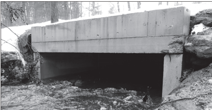
New culvert for Hayes Road over Dube Brook.
