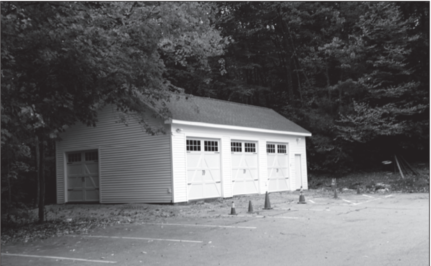
The new Building and Grounds shed.
