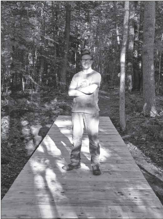
Sam Perley stands on a newly constructed boardwalk over a wet area, which was part of his Eagle Scout project.
