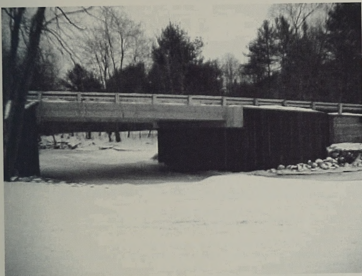
Sargent Hill Bridge – Photo by Steve Darrow
