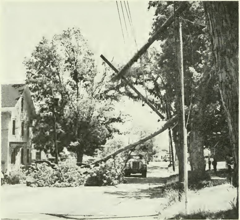
High winds caused this limb to fall bringing down cables and snapping off pole. Penacook CD Rescue Squad assisted Power Company employees at scene by roping off area, keeping pedestrians away, and directing traffic.
