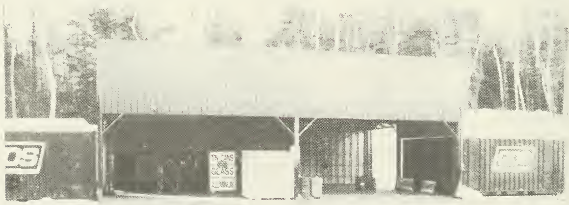
Wal-Mart provided funds for the Recycling Facility at the Transfer Station
