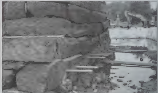
West face of pier: underpinning rods grouted in place
