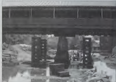
Temporary bridge tower supports
