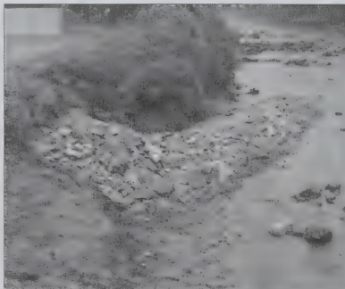
Completed west stream barb
