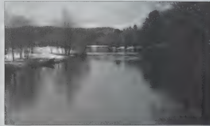
Looking upstream, beyond bridge, before dam removal
