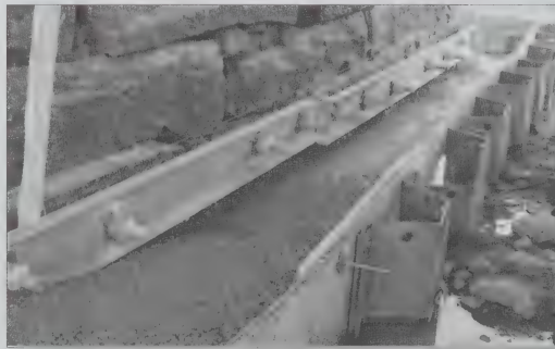
West face of pier: underpinning rods & channel, concrete placement
