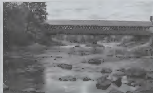
Completed project, looking downstream
