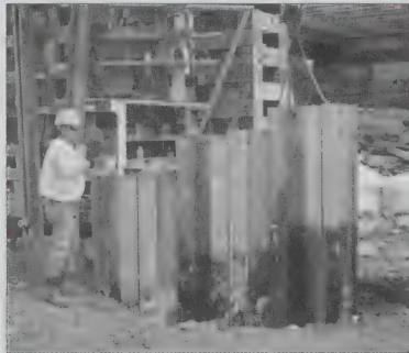
Installing sheet piling at center pier
