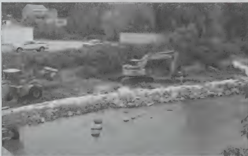
Constructing west stream barb
