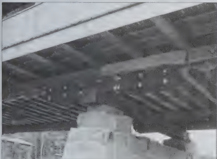
Re-installed pier sleeper beam
