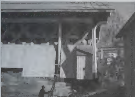
Sprinkler feed pipe at southwest corner of bridge
