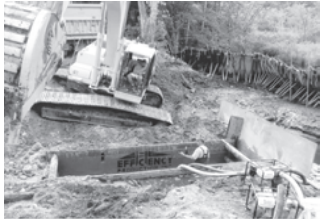
WORK GETS UNDERWAY ON THE SOUTH MERRIMACK ROAD BRIDGE AND CULVERT
