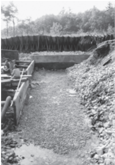
PREPPING FOR THE FOUNDATION
