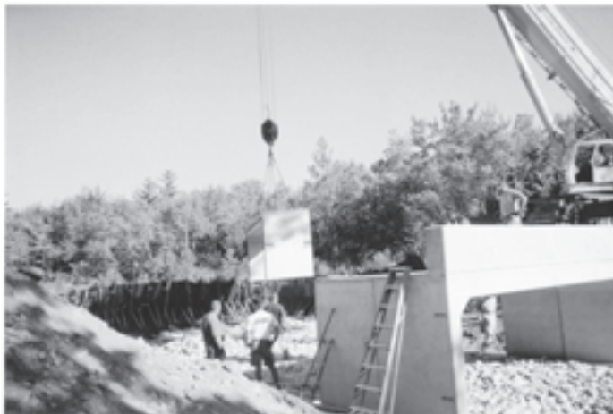
INSTALLING THE PRECAST CONCRETE
