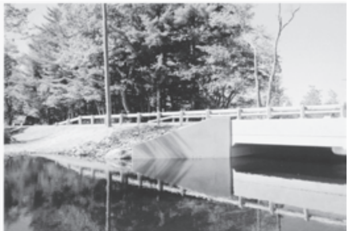
THE COMPLETED SOUTH MERRIMACK ROAD BRIDGE AND CULVERT
