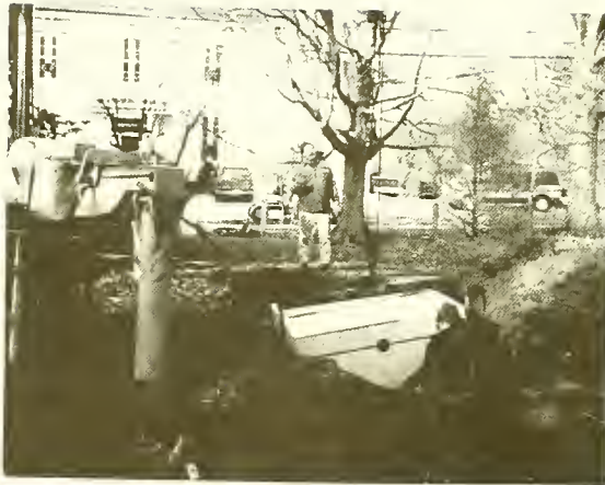
Septic system progresses
