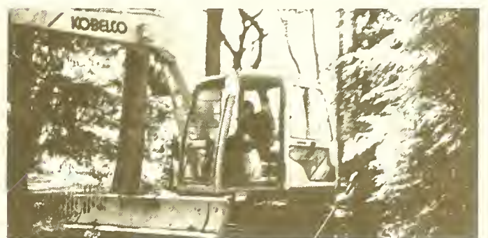
Covering water pipeline
