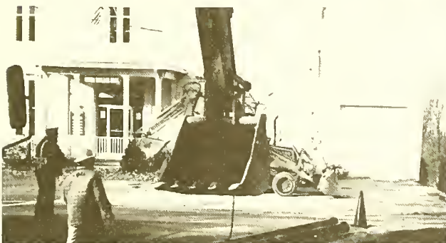
Excavating for Well & Septic Systems
