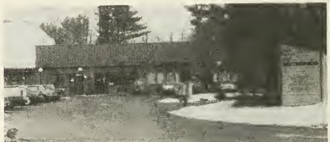
Metronics, Inc. a high-technology manufacturing firm received site plan approval for re-use of a building on Harvey Road.
