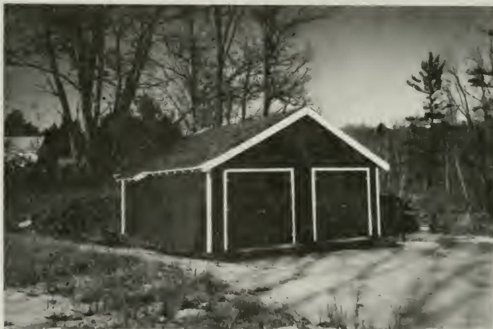
Alton's refurbished Parks & Playground/Highway Department storage building. This building set idle for years due to fire damage. Through the combined efforts of the two departments it is now being utilized.
