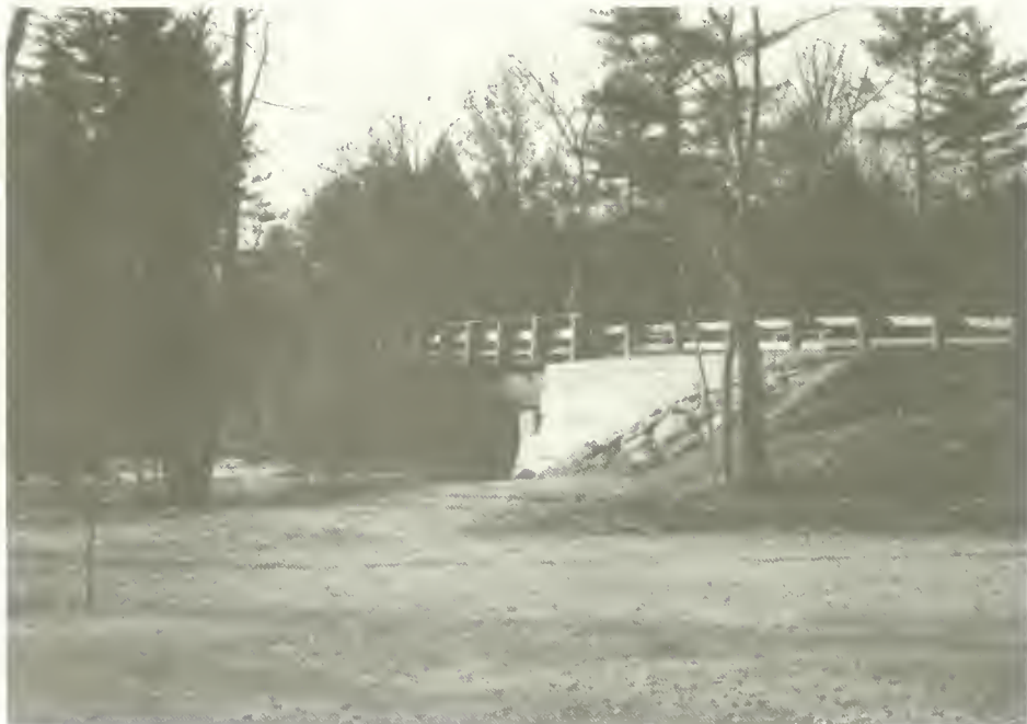
LINDEN STREET BRIDGE, 1993 (Following reconstruction)
