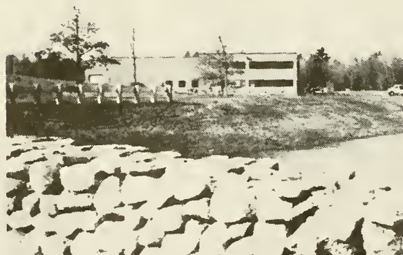
This new industrial site at Commerce Park West is one of the projects inspected for completeness by the Planning Department.
