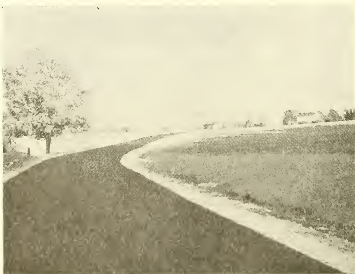
Curtis Road — After Reconstruction
