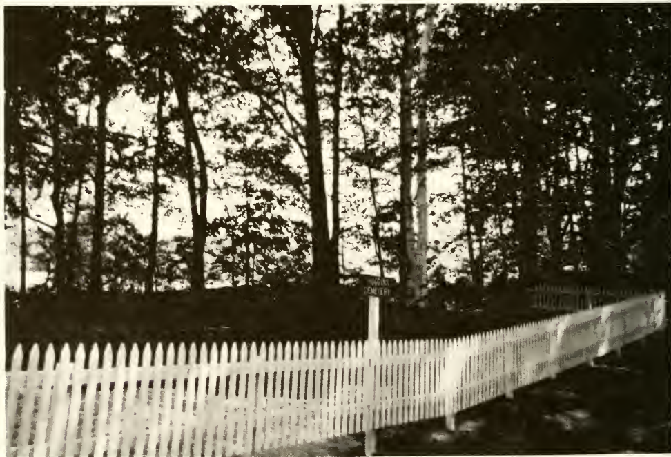
New fence around Huggins Cemetery
