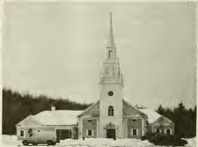
The Bethany Covenant Church under construction; reviewed and approved by the Planning Board in 1990.
