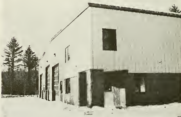
New Public Works Garage nears completion.
