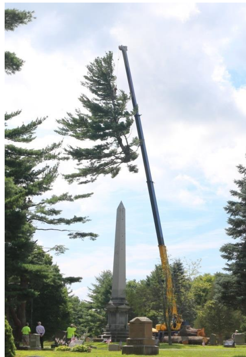
Crane removing the large unstable bull pine trees - August 2018
