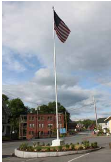
A full view of the newly restored Main Street flag pole. A 2009/2010 EVA project
